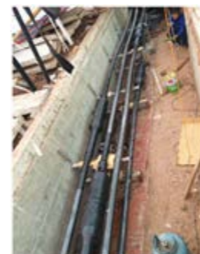
SK Chongqing Special Outside Substation Project
