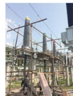
Sichuan Puge County Estuary Power Station Project
