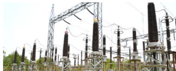
• 132kV CTEB-ET Dique-ET Tolosa Underground Cable Project in Argentina
