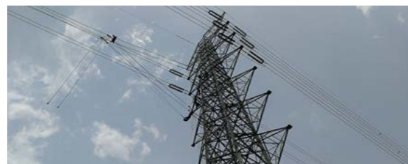
• 230kV&132kV Transmission Line for PGCB in Bangladesh
