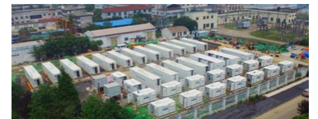
• Engineering, Procurement, and Construction of 20MW BESS Pilot Project in Pakistan
