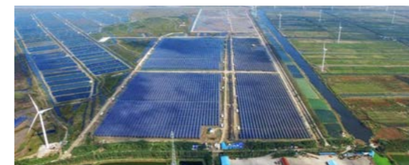
• Rudong 110 MW Photovoltaic Power Plant(BOO) in Nantong
