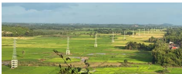
• 230kV&115kV Transmission Line for EDC in Cambodia
