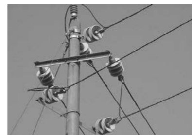
Dead-end for AAC conductor
