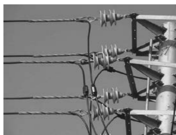
Dead-end for insulated conductor
