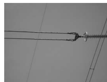
Dead-end for ACSR conductor
