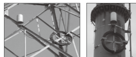
Installation on tower Installation on pole
